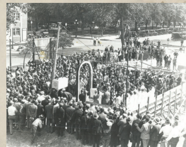
Laying the cornerstone at the Hastings Masonic Center on September 14, 1928
